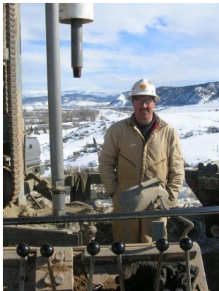
Joel managing geotechnical drilling operations.
