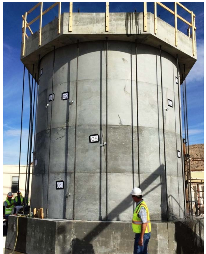
Testing a post-tensioned lining prototype for the L.A. Outfall Tunnel.
