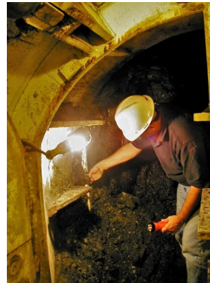
Rafael inspecting face of jacking operation at NBC CSO Program.
