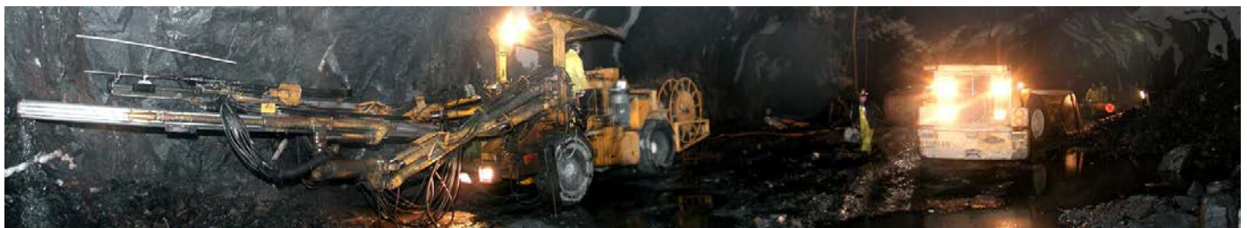
Blasting operations at NBC Pump Station Cavern.
